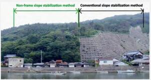
This technique stabilises the slope through the combination of natural approach and dan structural frame using plants and trees at the slope and the installation of several bolt stones (rod type of frame) along the identified slope areas.
