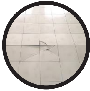
Buckled and cracked tiles
