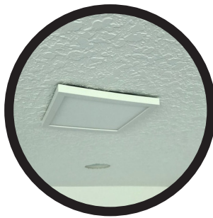
Gap between lighting and ceiling
