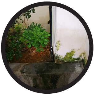
Mold on external wall
