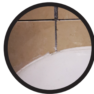
Inconsistent tile joints
