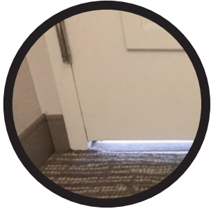
Excessive gap under the door frame
