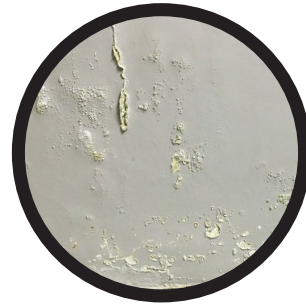
Efflorescence of paint
