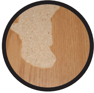
Peeling off laminate
