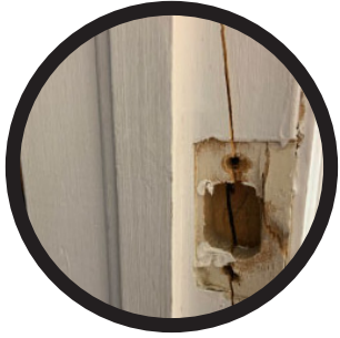
Cracks in door frame or panel
