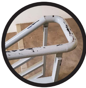
Paint peeling off hand rails
