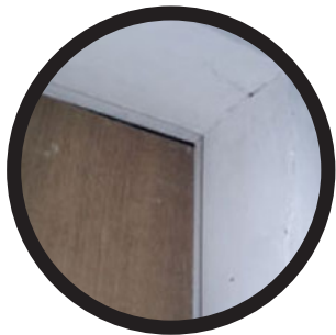
Buckling or Sagging of doors
