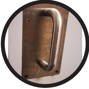
Rusted screws at door handle
