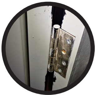
Missing screw at the door hinge
