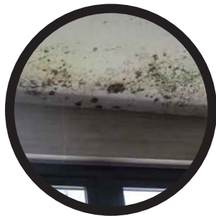
Water marks - mold found on ceiling finishes
