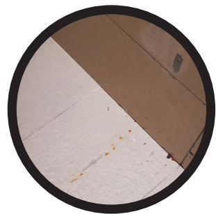
Rust stains on floor tile
