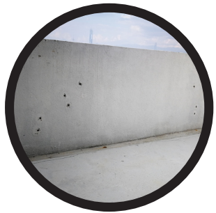
Parapet wall not properly touched up
