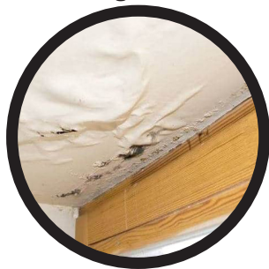
Sagging on ceillin plaster
