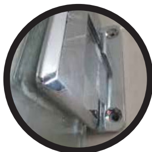
Screw at the shower screen found to be missing
