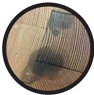
Timber floor Discolouration
