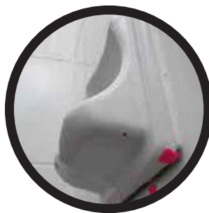
Visible gap around the internal fixture (soap holder)
