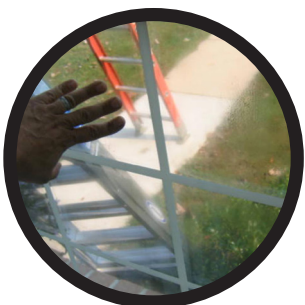
Condensation in double paned windows
