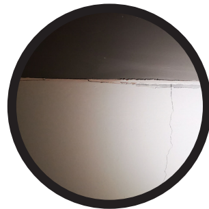
Cracked plaster ceiling
