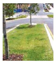
Bio-retention swale in a median strip
