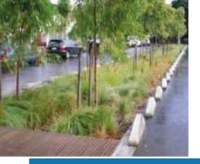
Kerb prevents access while the breaks in the kerb allow stormwater inflows
