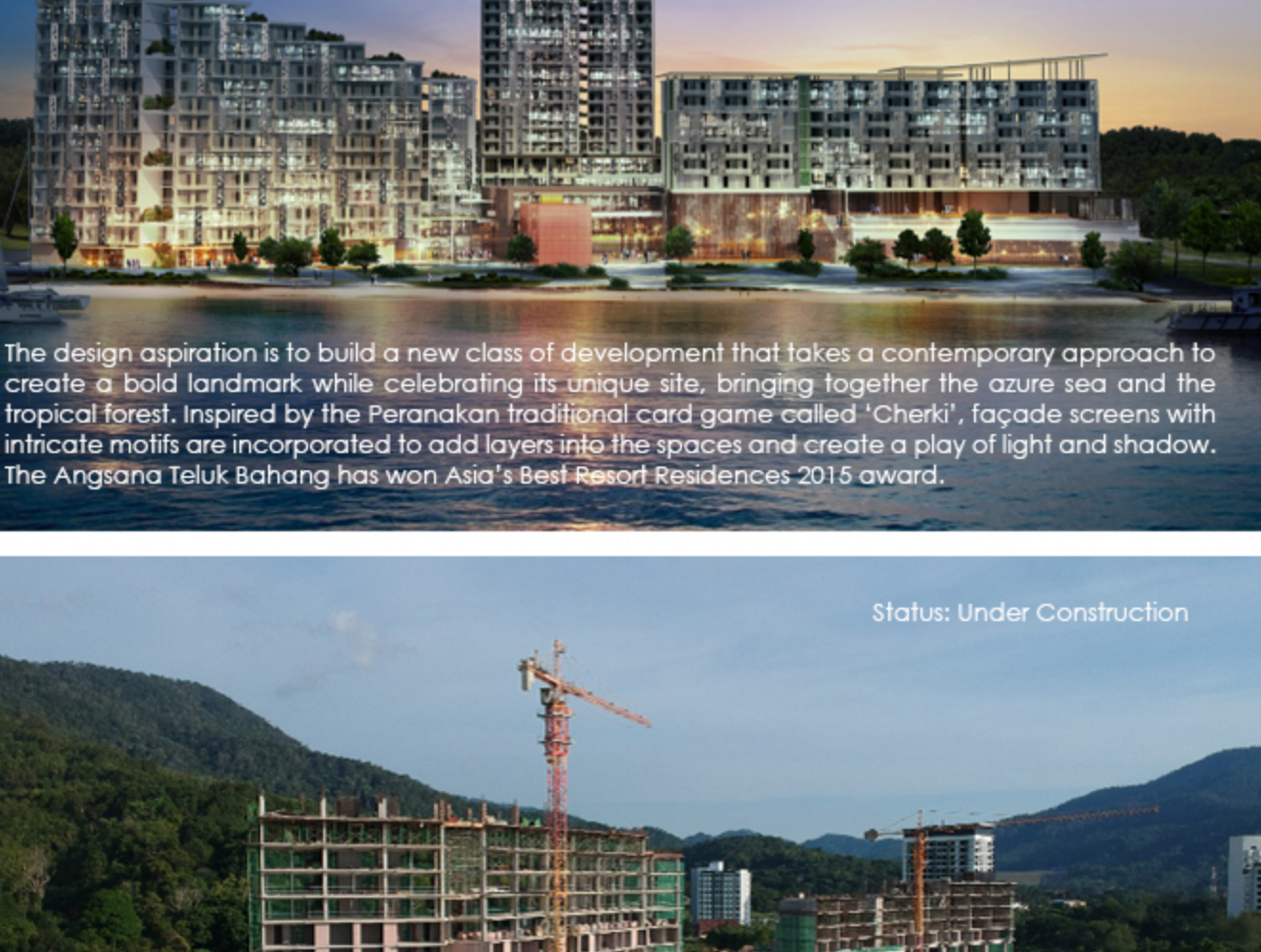
Status: Under Construction
