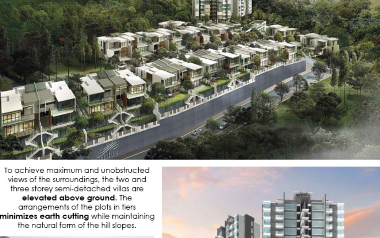
Status: Under Construction
