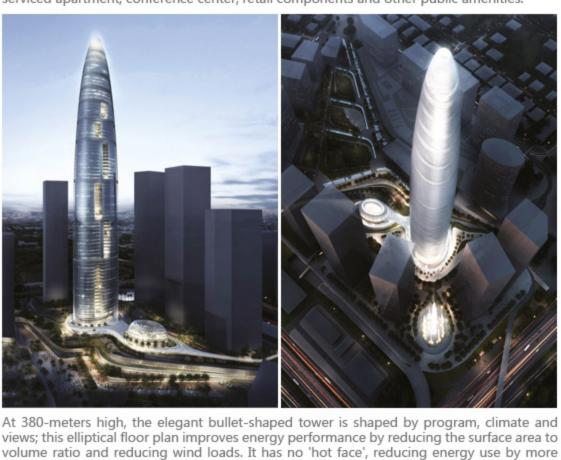
than 4% whilst producing 84% efficiency floor plans. The mechanical and structural engineering of the tower is optimized to allow maximum light penetration into the building. This tower is a model of fine-tuned efficiency that can be constructed rapidly, with significantly reduced materials and which will operate at LEED or GBI Platinum efficiency. YTL HQ, KUALA LUMPUR In collaboration with Kohn Pederson Fox Associates, United States of America
