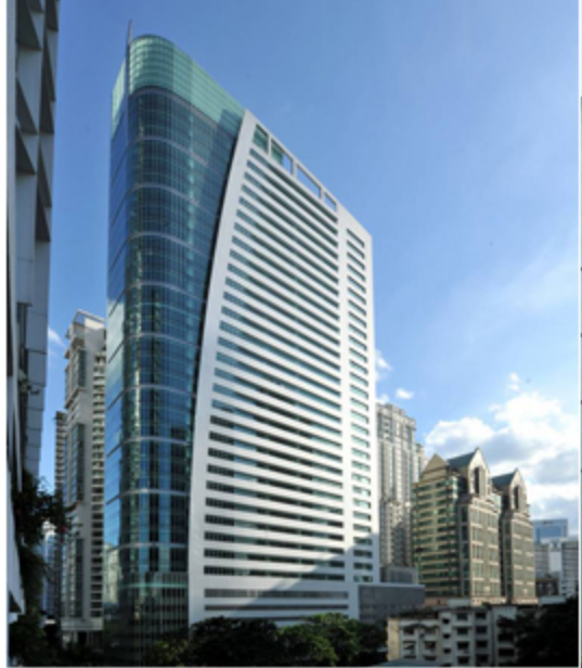
To achieve a wider frontage, the entrance is placed at the longer side of the building and is further denoted by advertisement billboards on the podium.
